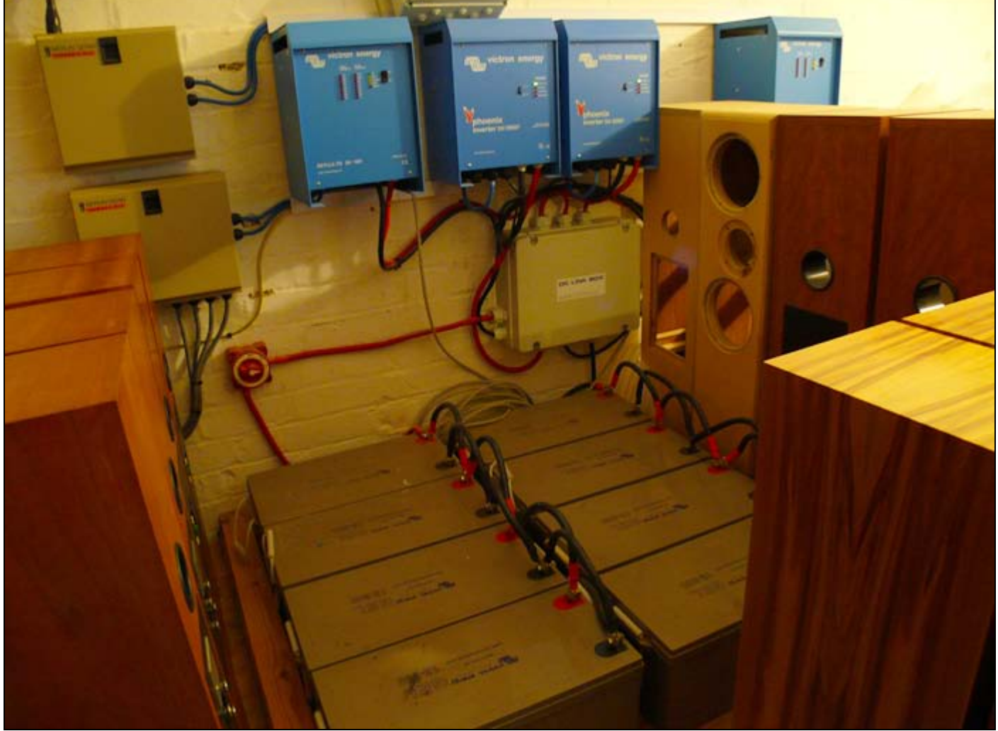
Ensconced by reject cabinets, the Definitive Audio loft contains this massive battery bank to run entire systems off the grid.
