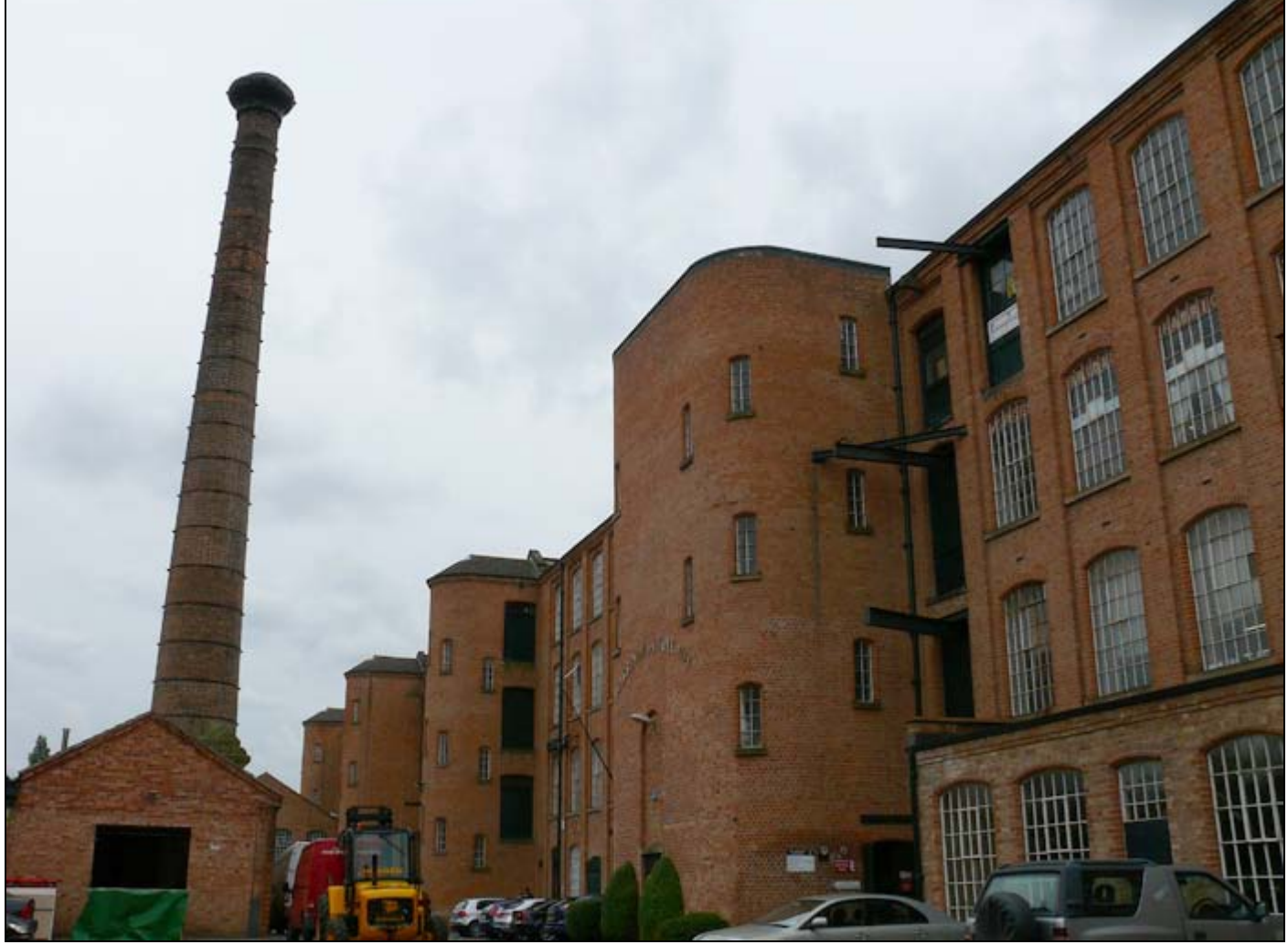
The tall chimney makes for quite the landmark.
