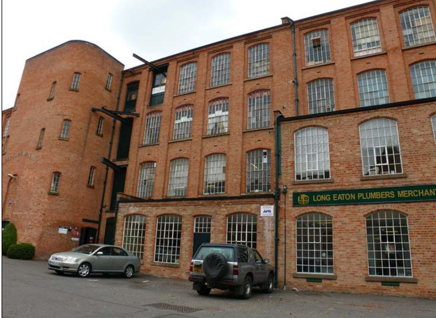
The Harrington Mill complex is a sizable industrial affair.
