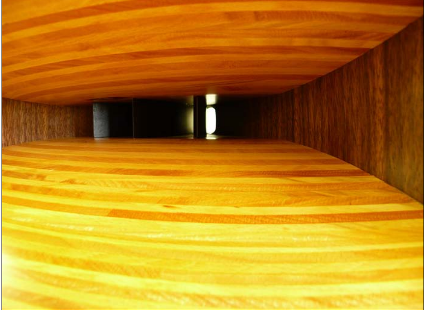
The short vanes in the throat of the midrange horn.
